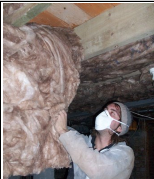
South Seeds handyman, Uillie, installing under floor insulation.
