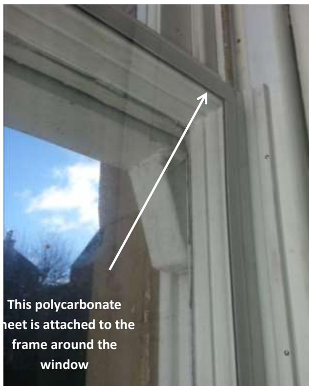
This polycarbonate sheet is attached to the frame around the window
