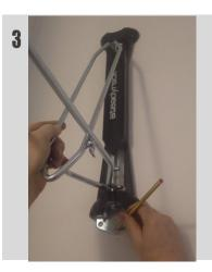
Mark attachment points for the rack Position the top of the wheel-support rack level with the mark on the wall and at least half the width of the handlebars away from any other object. Ensure the rack is straight with a spirit level and make marks on the wall where the attachment holes are.
