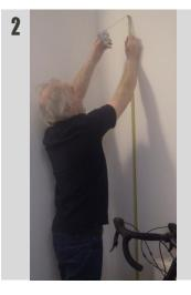
Measure your bike Measure the length, add 10cm and mark this measurement on your wall from the floor. Also measure the width of your handlebars.
