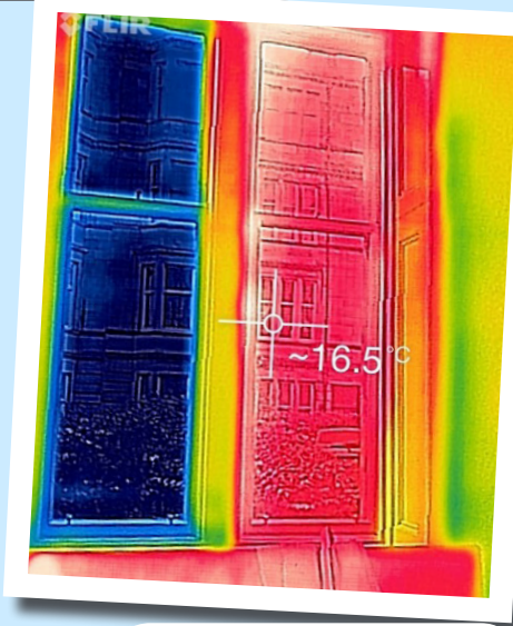
A thermal image of heat-retaining polycarbonate glazing
