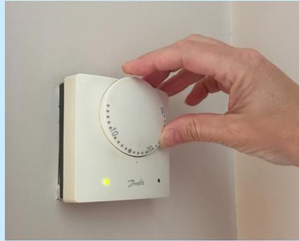
Most room thermostats are fixed to a wall in a draught-free area, and only work when the central heating is turned on – at the boiler switch or via a timer.
